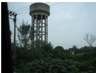
Figure 12.3.1 Overhead Service Reservoir
