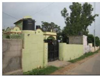
Figure 12.3.2 Overhead Water Tank
