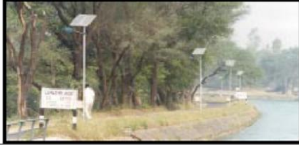
Figure 12.4.5 Solar Panels for street lights
