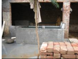
Figure 12.3.4 Ground Level Water Tank
