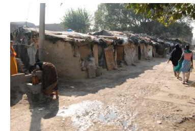
Dilapidated houses at Slums
