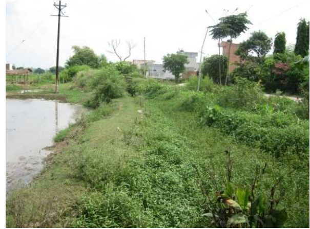
Fig No. 52:- Distributory is full of weeds, shrubs and domestic refuges instead of water supply near ITI Institute
