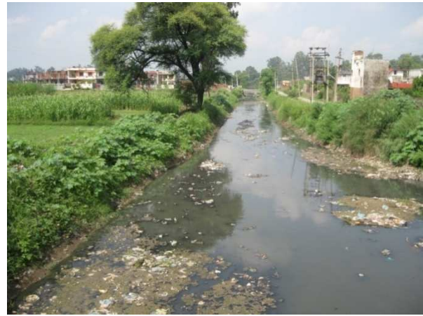
Fig No.56: Drain becomes the dumping sites of domestic refuges and biomedical waste at Hargobindpur Mohalla.
