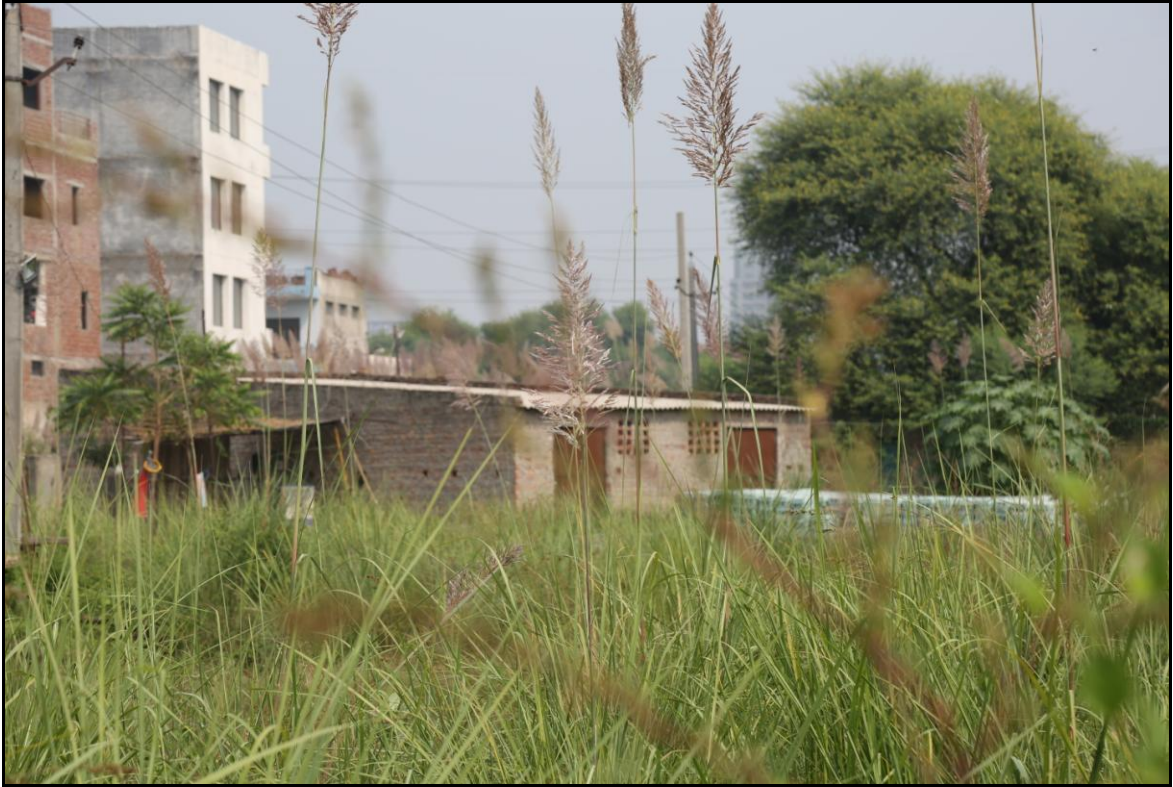
Structure in proposed land acquisition
