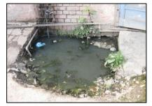
Fig no.87: View of Blocked Sewer at Mahan Singh Gate
